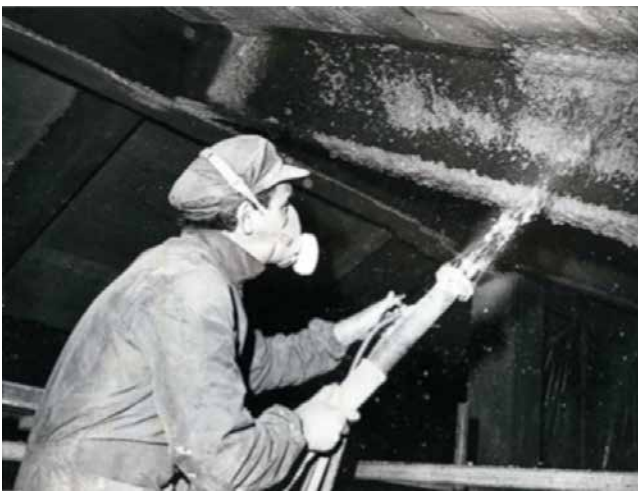
Thermal Insulation Engineer applying fire protection to structural steel.
