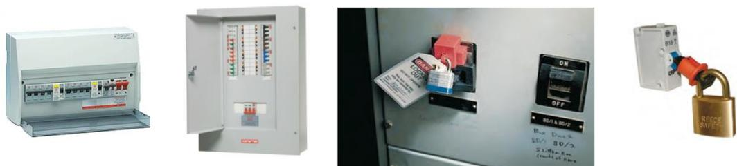
Figure 1 – distribution boards and disconnectors
