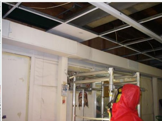
07/08/23 11:30 Final tile that was awkward to remove.
