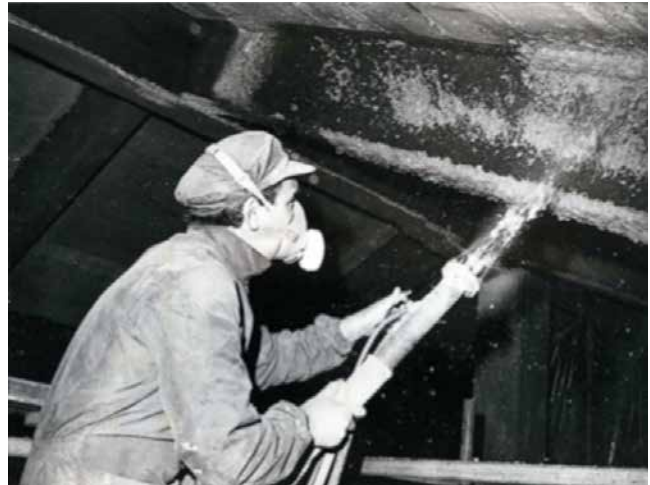
Thermal Insulation Engineer applying fire protection to structural steel.
