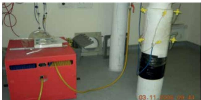
This picture shows a system commonly known as 'the red box'. The pipe work to the right is being injected with the wetting agent prior to removal. The injection needles can be clearly seen protruding from the pipe.
