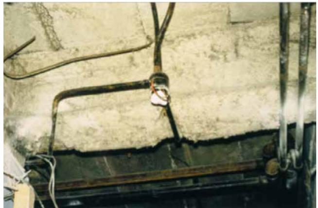
*Sprayed coating applied to structural steel. Note the damage around the electrical junction box.*
