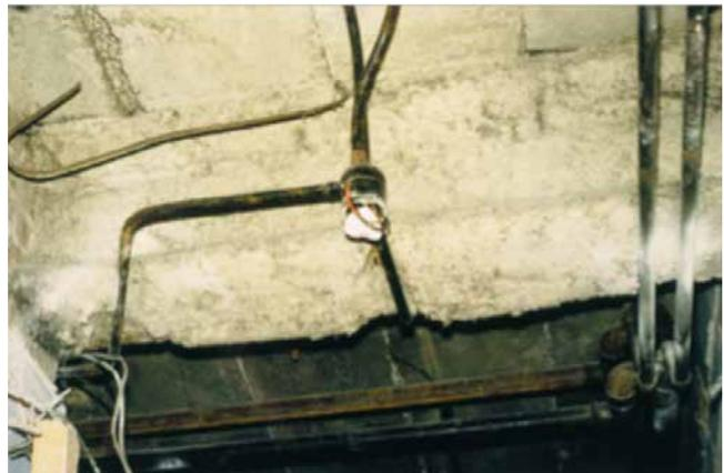
*Sprayed coating applied to structural steel. Note the damage around the electrical junction box.*
