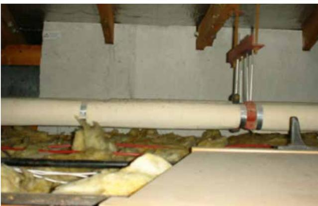
AIB as a firebreak in a ceiling void.
