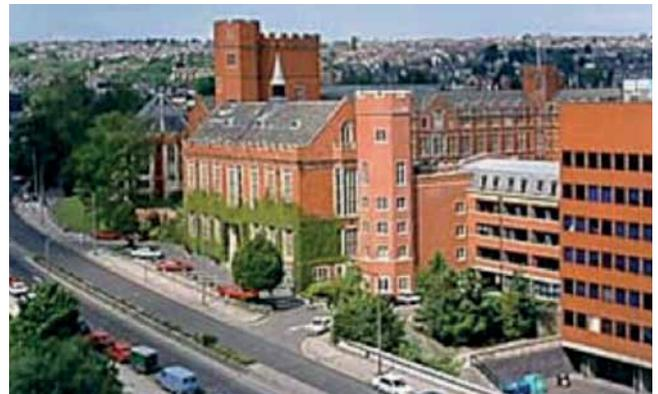
Early 1960s steel, glass and concrete with steel framework with potential sprayed asbestos applied. Internal lifts could be lined with AIB and a sprayed coating applied to the large foyer area.
