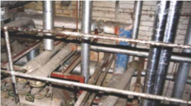
Thermal insulation can come in many forms such as hand applied thermal lagging used for pipe and boiler lagging.
